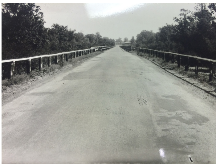
The Angelina River Bridge at the county line when it was still SH 35.
